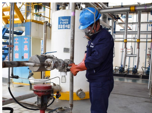
Shandong Huahong has installed flanged sampling valves on its process pipeline and tank openings to reduce risks to staff performing sampling work
